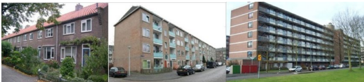
The three building typologies that are included in the Dutch 111,000-deal. The prototypes for the first type (terraced houses) and second type (4 story buildings) have been delivered (700 in total by Q2 2015). The multi-story flats will be prototyped later in 2015.
