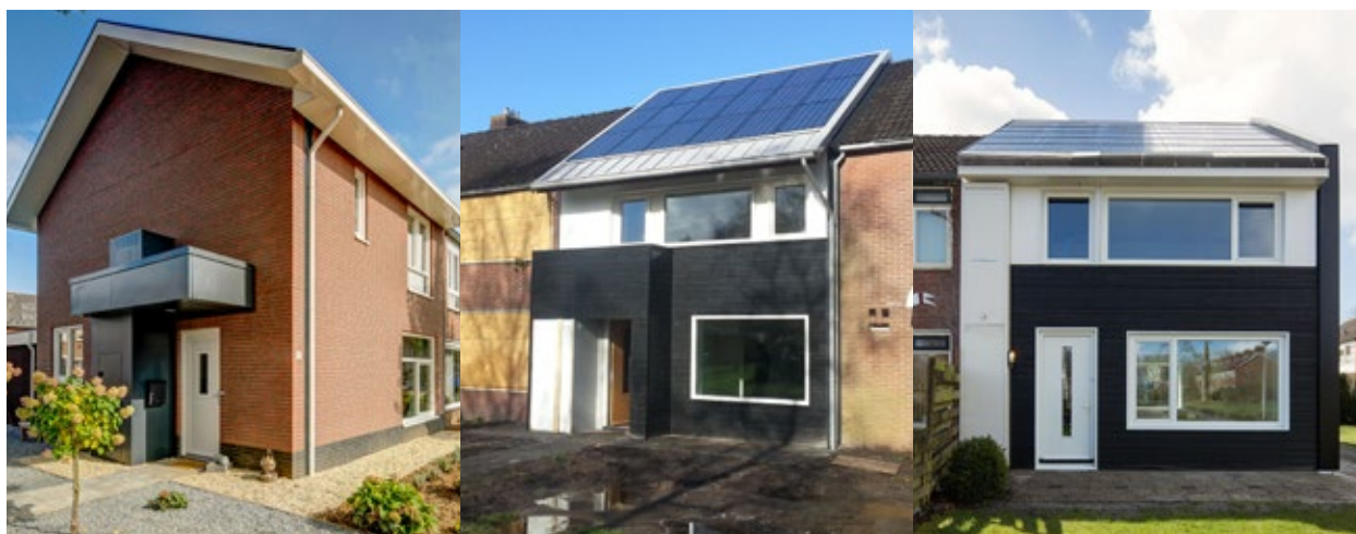
Three prototype versions from one company (Volker Wessels): Version 1, (Dec 2013, left) took 2 weeks to place and has the energy module sticking out; version 2 (middle) took 1 week and has the energy module more integrated around the front door. Version 3, (February 2015, right) took 1 day and has the module integrated in the façade. Cost reduction between version 1 and version 3 is \pm 30\% . Watch the movie of the 1 day refurbishment here: https://www.youtube.com/watch?v=I3WBT2eAArI
