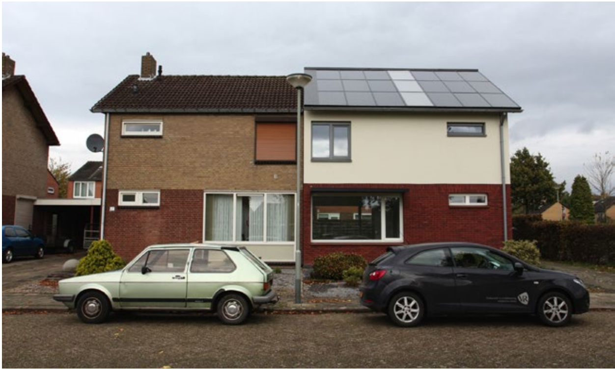
Roll out of an E=0 refurbishment with 30 year guarantee
